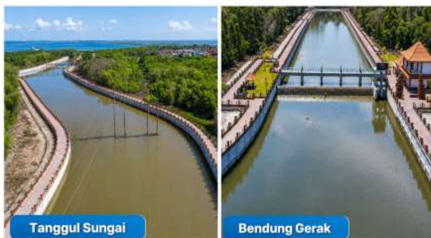
Figure 3. Long Storage Tukad Mati Infrastructure – River Embankment (left) and Movable Weir (right)
