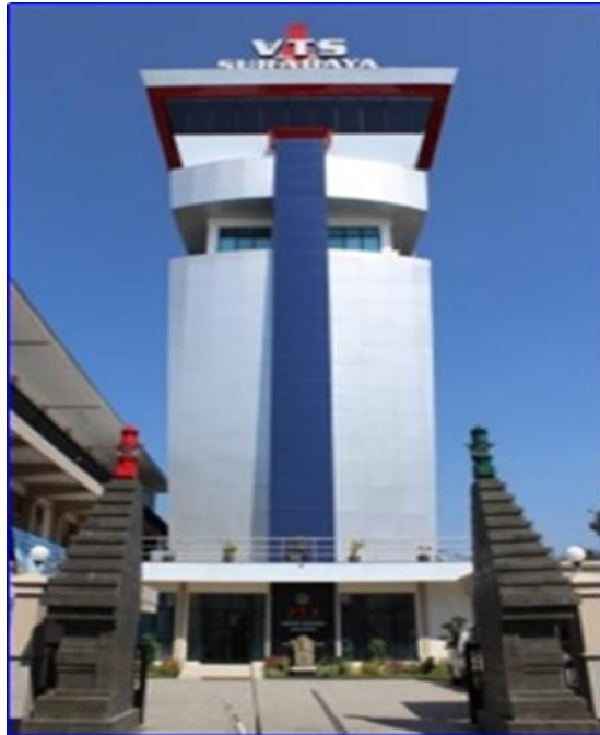
Figure 1. VTS Building of Navigation District Class I Tanjung Perak Surabaya
